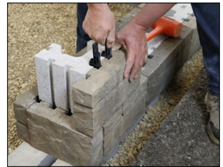
Diagram 22—Wall end example
