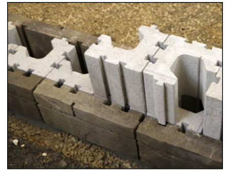
Diagram 21—Second course construction
