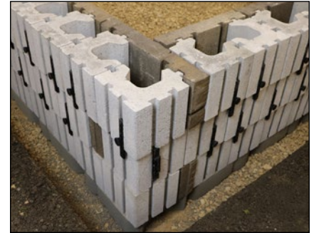
Diagram 12—Corner unit formed
