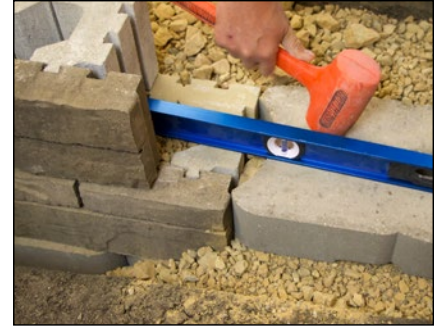
Diagram 7—Stepping up the base
