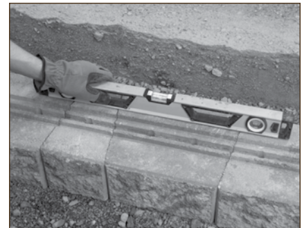
Diagram 2 - Level each unit
